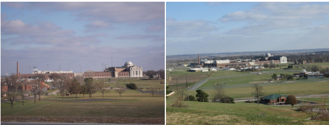
Photos 6, 7: Views (looking eastward, including from Santa Fe Trail) of West Site with Existing USP in Background
