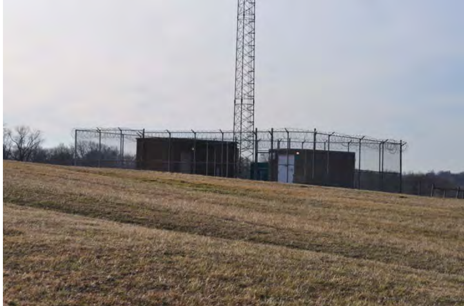
44_Cell Tower and Bldgs South of Dairy Barn_View SE.JPG
