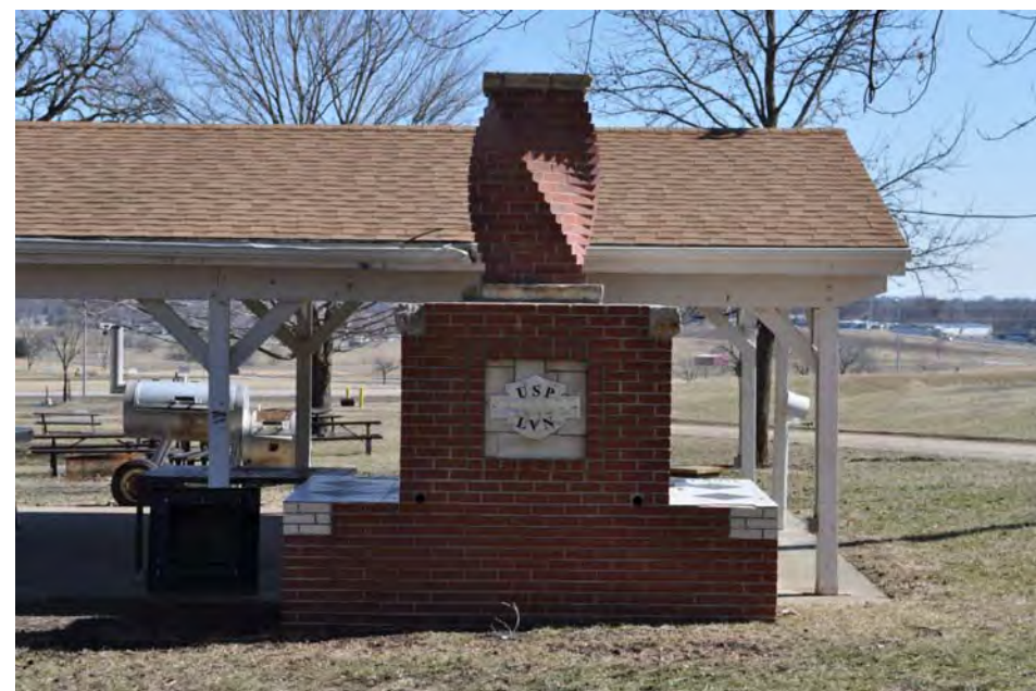
54_Brick Grill in Picnic Area_View SE.JPG
