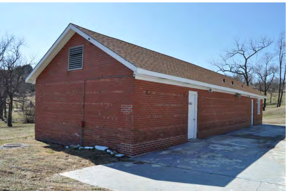
49_Toilet Block_View SW.JPG
