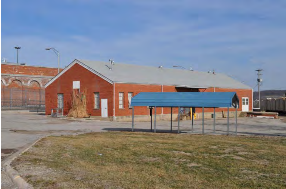
28_Receiving Depot_View NW.JPG
