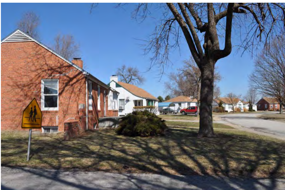
Staff Housing Overview_View N.JPG
